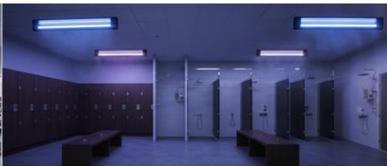
UVC mode: Full disinfection cycle activates automatically when unoccupied
